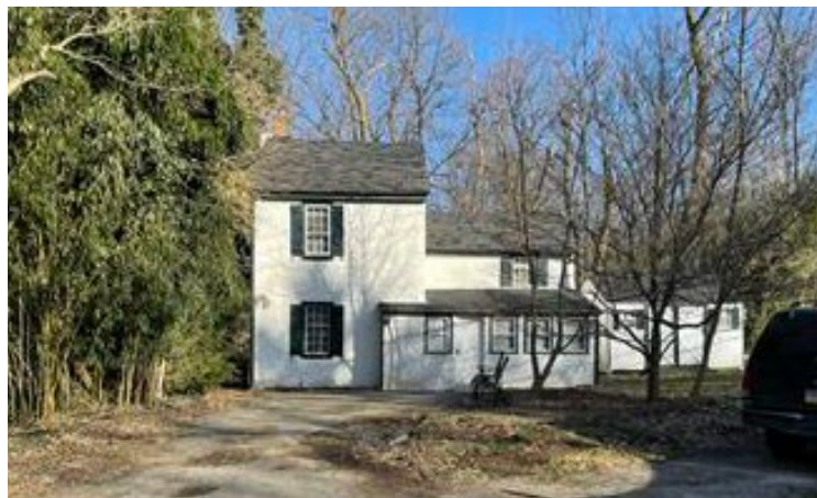
Halfway House (011). Built in 1833 by the West Chester Railroad Company (Commonwealth 2021).
