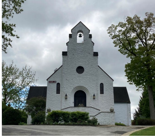
Chapel of the Atonement (025.07) at the Church Farm School (Commonwealth 2021).
