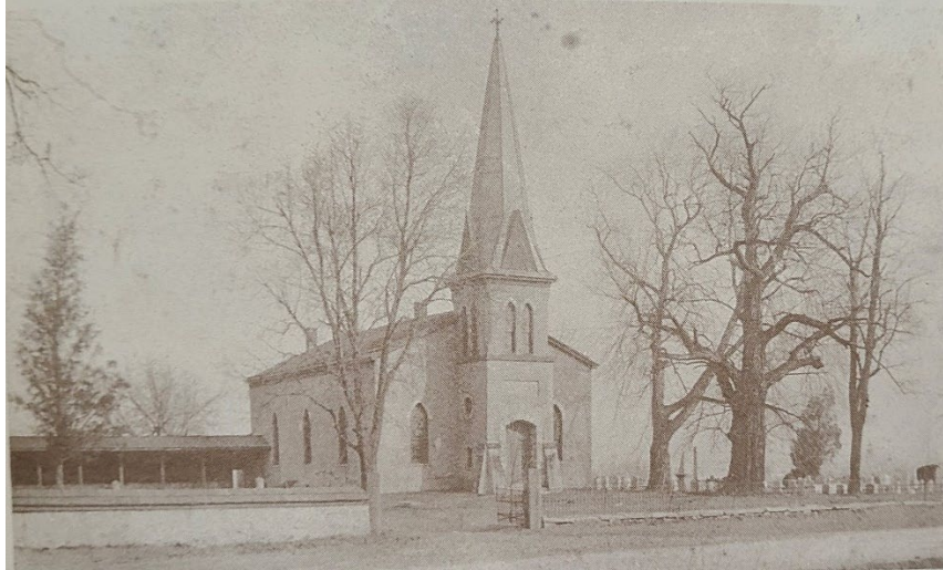
St. Paul's Church (347) c. 1900. Horse sheds on the left were replaced by a Parish house in 1912. Note the dirt packed Route 30. Courtesy of St. Paul's Church.
