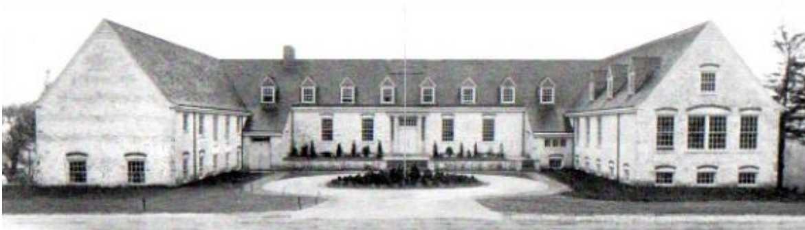
Greystock Hall (025.01) at Church Farm School as it appeared in 1935 on a traffic-free Route 30. Courtesy of Dr. Charles W. Shreiner, Jr.
