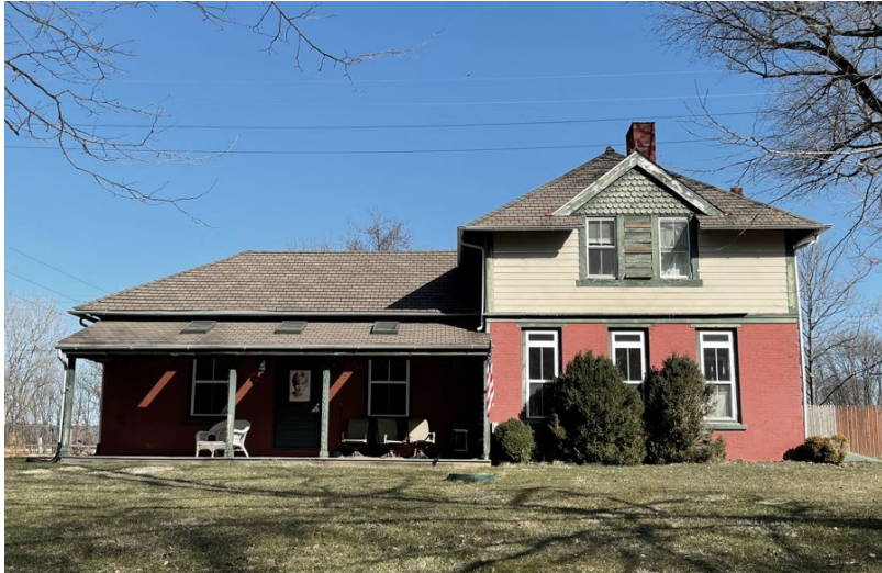
Glen Loch Station (023) built c. 1890 (Commonwealth 2021).
