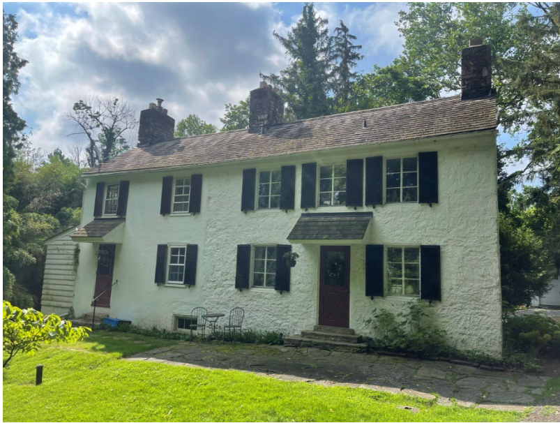
Wee Grimmet (123) constructed c. 1820 as a worker's cottage for a local quarrying and limekiln operation (Commonwealth 2021).
