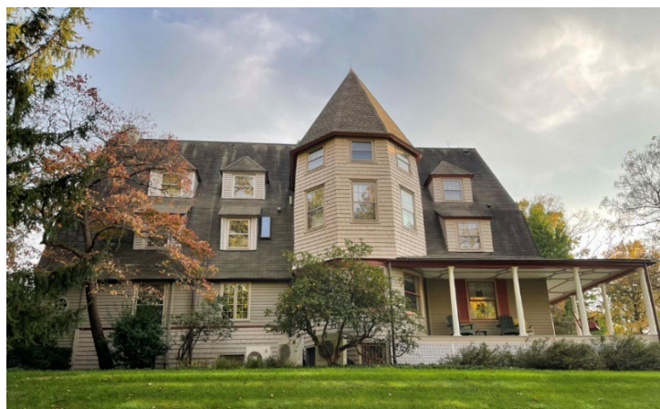
Francis W. Kennedy House (143). Designed in 1889 by renowned architect Frank Miles Day as a summer cottage in Bradford Hills (Commonwealth 2021).
