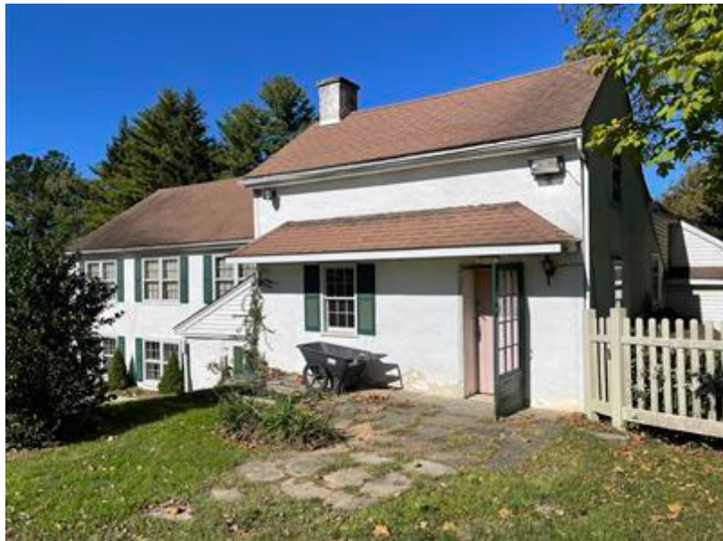
Office and Quarry Master's House (103.03) for Thomas Marble Quarry (Commonwealth 2021).
