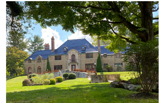
5.15, 5.16. The tile roof of a Class II Historic Resource in Wynnewood was replaced with a solar tile system despite the HC's determination that the change was inappropriate.
