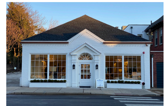
5.6, 5.7. The brick facade on Haverford Station Road, before and after being painted by its new tenant. The project also included improvements to the entry surround and storefront windows that HARB reviewed favorably.
