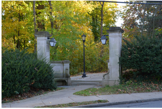
3.7. The Conklin Memorial Gateway on the Haverford College campus would likely qualify for Class I designation. It was an early work of pioneering African American architect Julian Abele.
