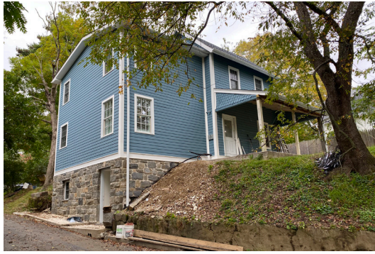
5.11. Smith Cottage during renovations.
