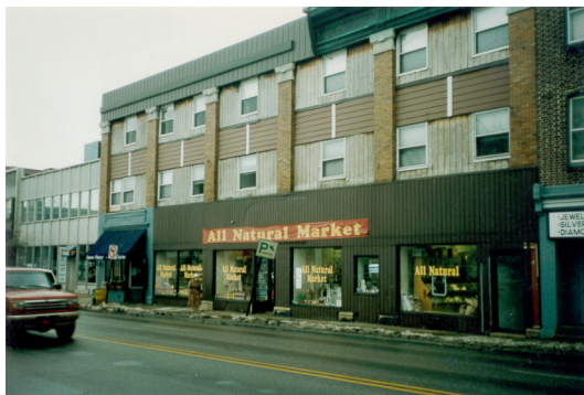
1.7, 1.8, 1.9. Three views of buildings within the Ardmore Commercial Center Historic District in the mid-1990s, shortly after the establishment of the District.
