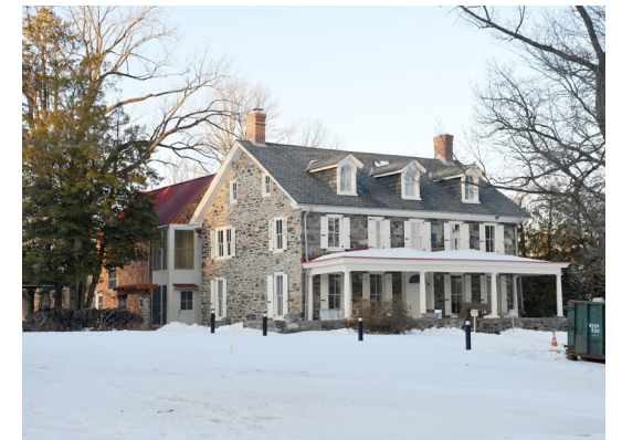
1.18. The HC reviewed modifications to Ashbridge House, including a large rear addition, prior to New Horizons Senior Center's occupation of the building in 2026. The house contributes to the Class I property and the work was managed by the Township's Parks & Recreation Department. The HC's consultation on various aspects of the project was essential to its success as an appropriate alteration.
