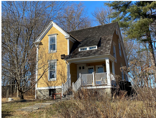
1.14, 1.15. The cottage at Rolling Hill Park, designed for the estate of Irwin Megargee, before and after restoration by the Lower Merion Conservancy.
