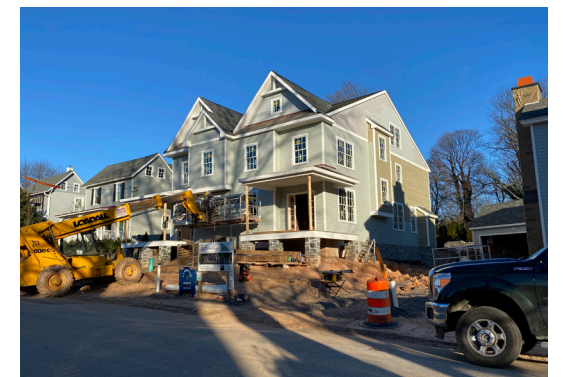
4.11. Heritage at Haverford was an economically viable project thanks to the construction of a new twin residence between two historic homes within the Haverford Station Historic District. The moving of one of those homes to the edge of the lot, using form relief incentives via Conditional Use, created space for the new construction.
