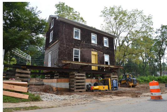
5.3. The historic house at 503 Old Lancaster Road being moved to a new foundation at the end of the parcel.
