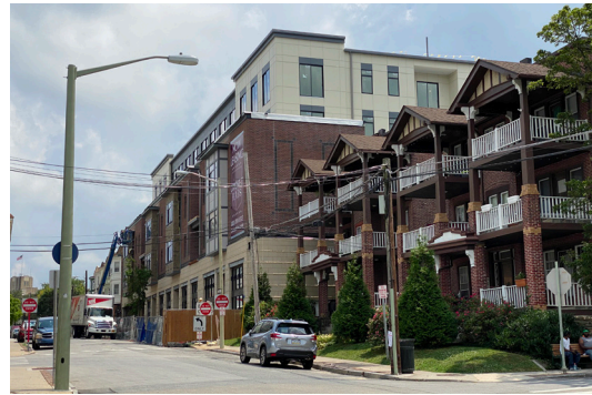
5.1, 5.2. The demolition of contributing buildings within the Ardmore Commercial Center Historic District (above) allowed for the construction of the Cricket Flats mixed-use development (below).
