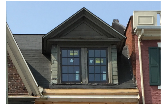
4.14. The center horizontal muntins of the modern replacement windows in this dormer window found in the Ardmore Commercial Center Historic District were made thicker to replicate the appearance of a meeting rail. Even though an egress-compliant casement window will not replicate the visual depth of a double-hung window, design choices like this can help a replacement window retain proportions and a visual link with historic windows.
